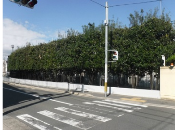
After exterior wall renovation
