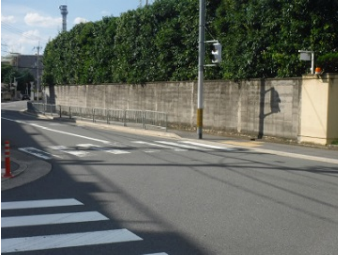
Before exterior wall renovation
