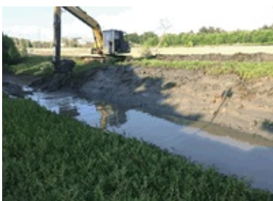
River dredging work (SGS)
