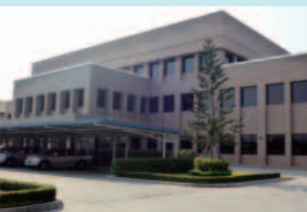
Head office of Siam GS Battery Co., Ltd.
