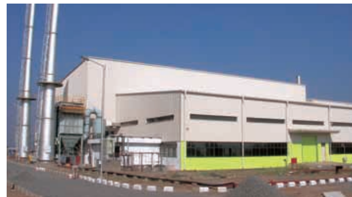
▲工厂全景 Overall image of the plant
